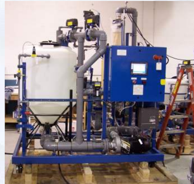
Field Evaluation ASCF for Primary concentration & high volume processing 7.5 – 38 m 3 /day
