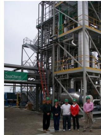
Figure 22: ZeaChem demonstration facility under construction, September 2011.
