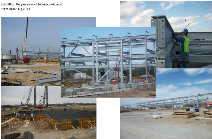
Figure 12: Myriant construction progress March 2012.
