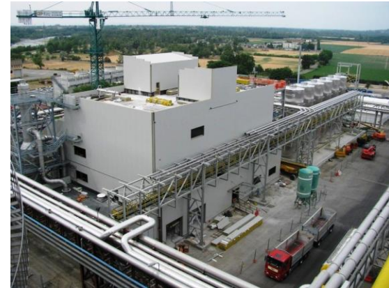
Figure 17: Reverdia commercial plant under construction June 2012.
