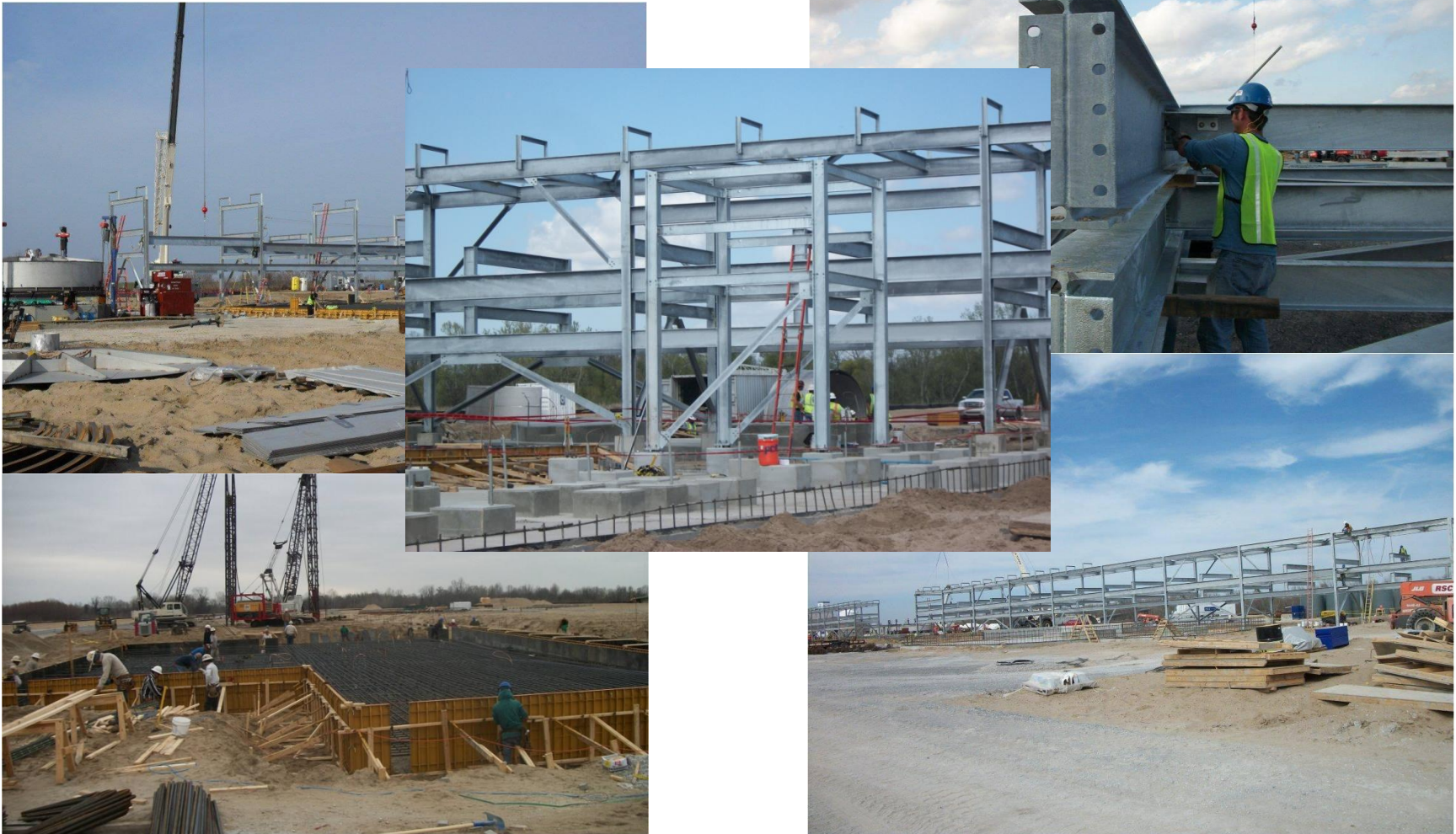
Figure 14: Myriant construction progress March 2012.
