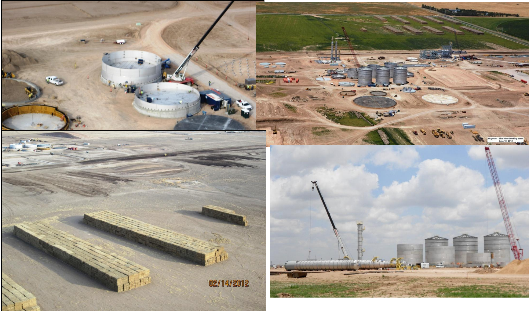
Figure 1: Abengoa biorefinery project stack yard.
