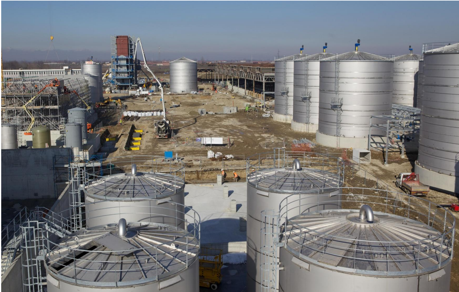
Figure 3: Beta Renewables construction progress July 2012.
