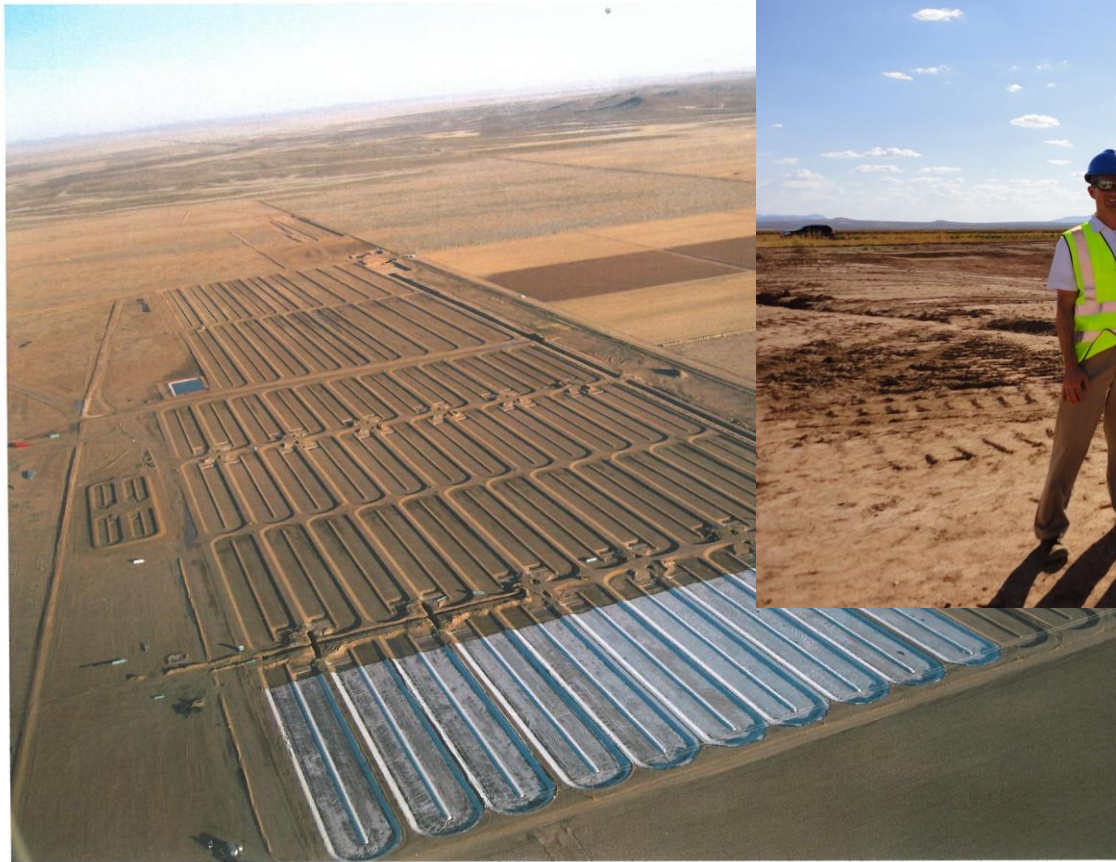
Figure 20: Sapphire IABR construction progress November 2011.
