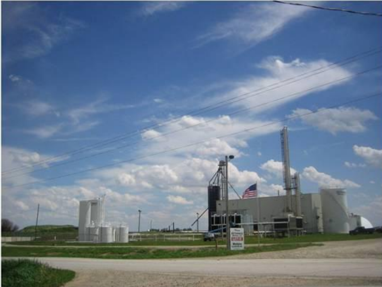
Figure 10: Fibright biorefinery undergoing renovation to cellulosic ethanol April 2012.
