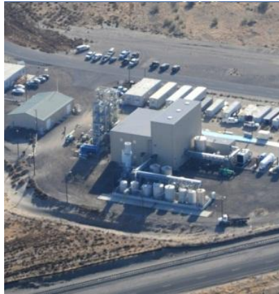
250K GPY Demo Facility Boardman, OR
